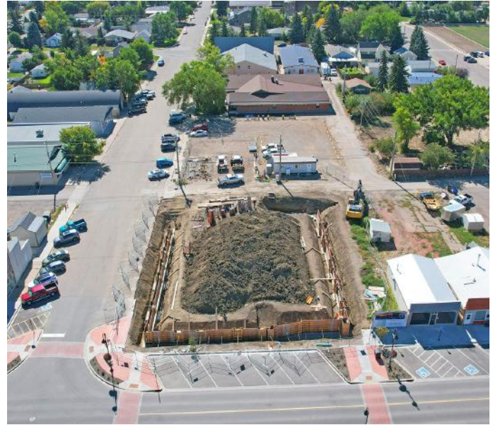
Shot of the build site looking South over Coaldale.
